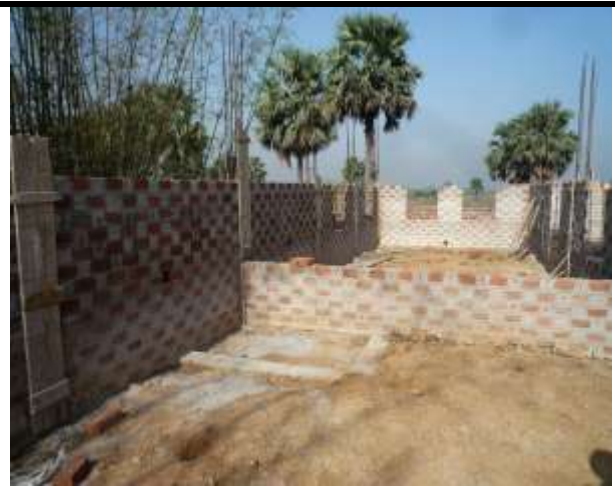
Rooms taking shape
