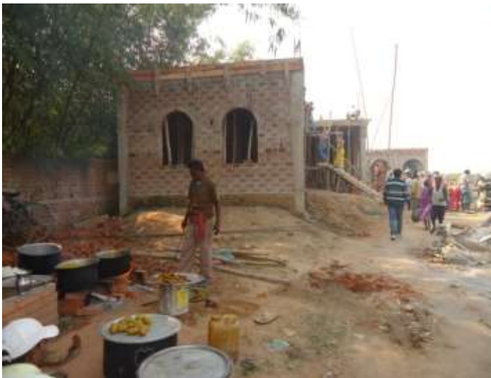
The roof goes on – November 2014
