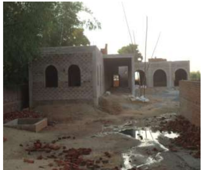
The verandah in place – February 2015
